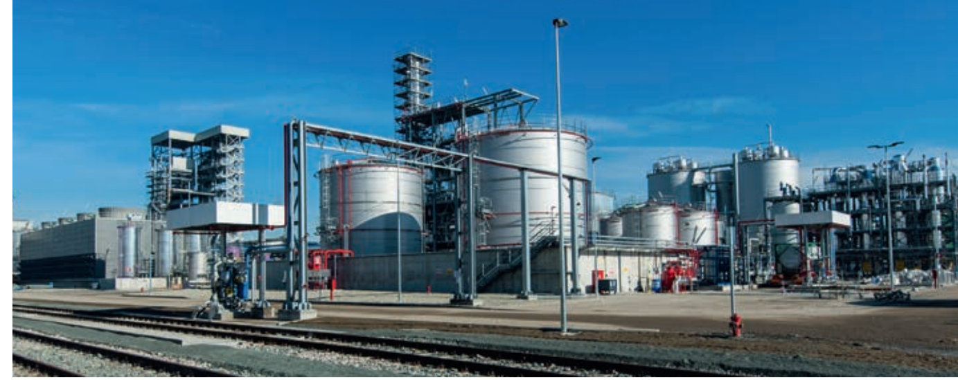
Plant in Crescentino (Italy)
